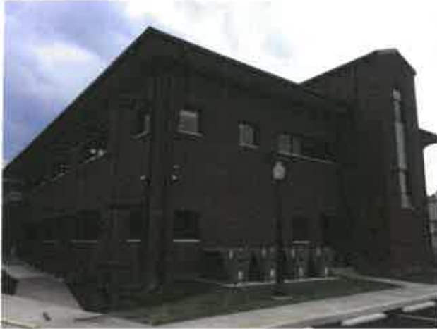
DISTRICT 1 OFFICE BLDG.
