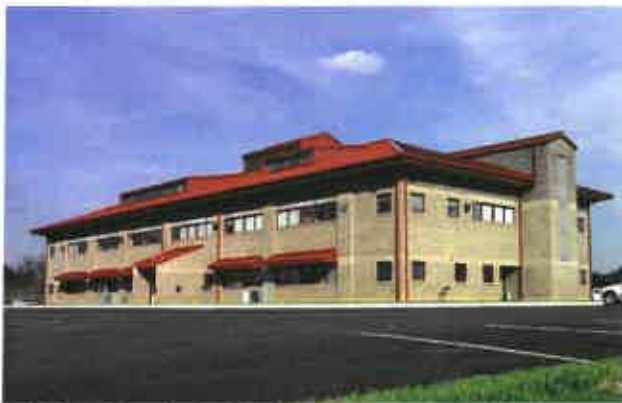
DISTRICT 10 OFFICE BLDG.
