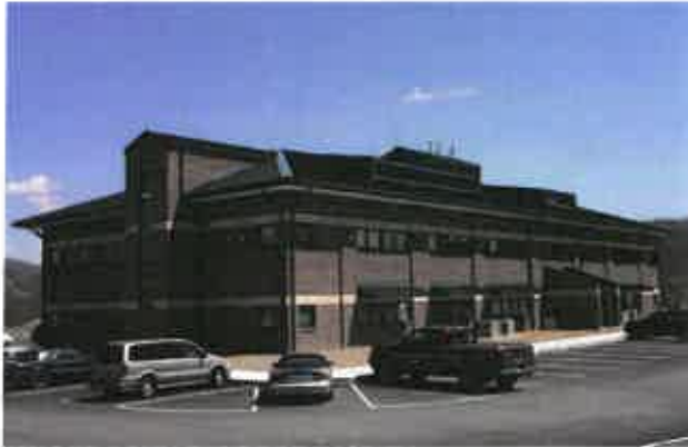
DISTRICT 6 OFFICE BLDG.
