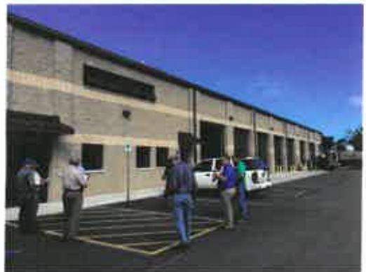
DISTRICT 8 EQUIPMENT SHOP
